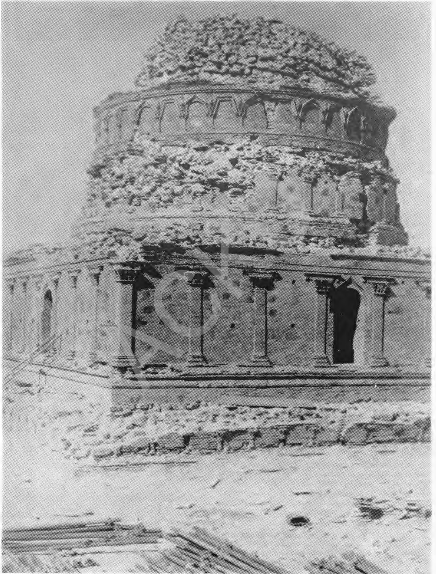
The northern part of Guldara's stupa after being repaired.
